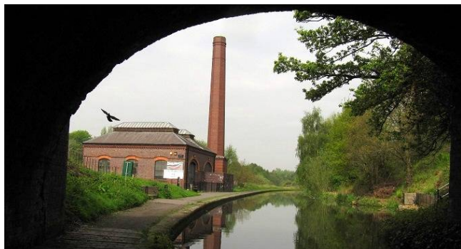
Galton Valley Pumping Station
