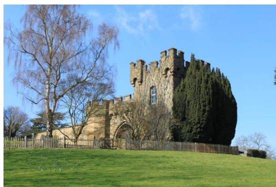
Arley Castle remains in local sandstone
