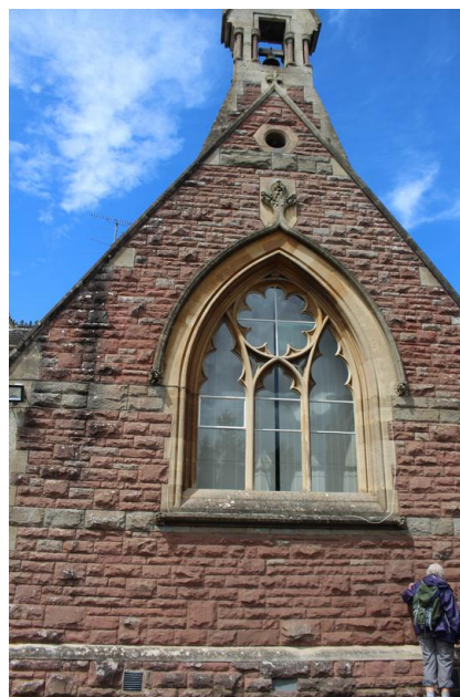
Bromsgrove Sandstone and Bathstone used in Huntley Church
