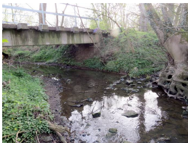
Fig.7. Loose blocks of dyke rock in Coatham Beck, near Eaglescliffe
