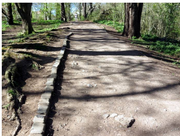
Fig.8. Cleveland Dyke edgings along the paths through Eaglescliffe Woods
