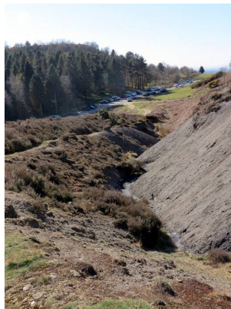
Fig.15. A muddy stream bed on Ayton Banks, with evidence of the dyke
