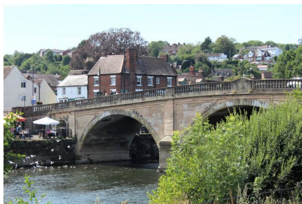
Bewdley Bridge, made of Carboniferous Highley Sandstone, and a red Triassic Sandstone
