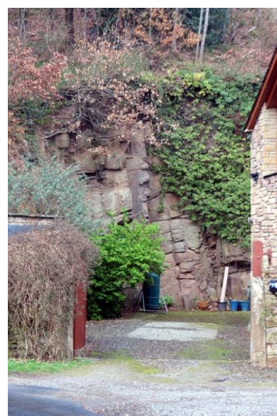
Fig.5. Crook's Mill Cottage: box-jointed Armathwaite Dyke
