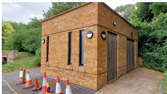
Fig.9. The new toilet block by All Saints Church
