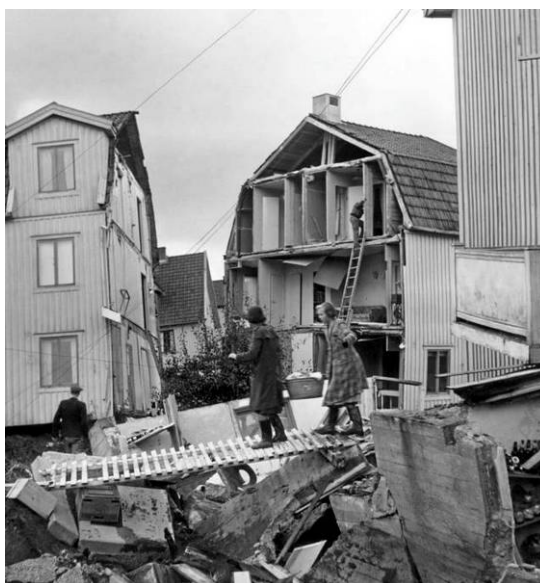
Surte, Sweden 1950. The landslide has split the house in two! Wikimedia Commons
