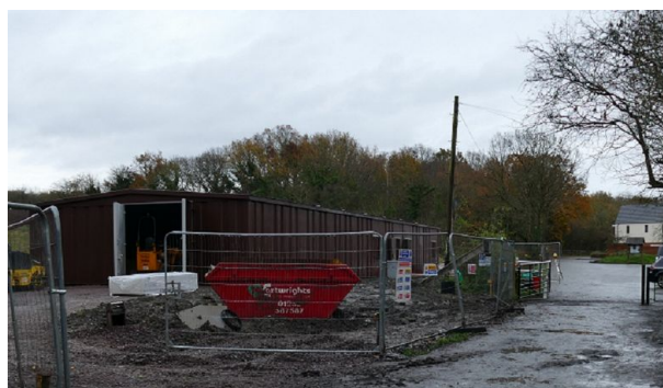
Saltwells Wardens' Base nears completion
