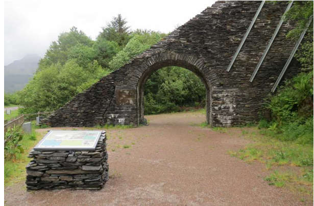
The magnificent slate arch, partially restored
